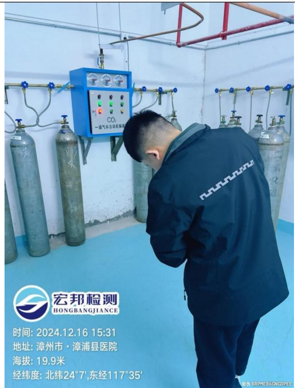
拟建DSA机房正上方机房
